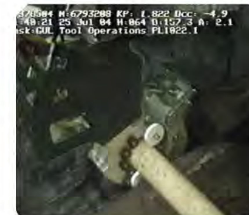
First sub-sea inspection.
