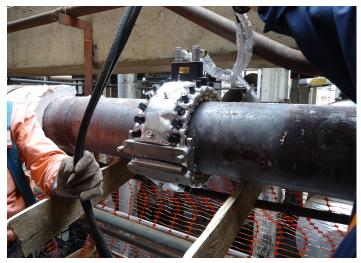
An 8" diesel line operating at 240°C (or 464°F)being tested by a HT inflatable ring.
