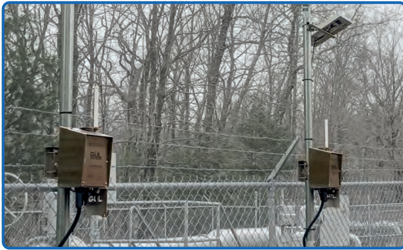
Solar-Powered FCUs – connected to sensors installed on buried pipelines
